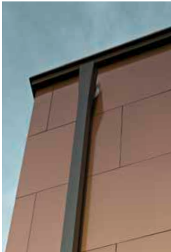
PREFA square downpipe with parapet outlet connector
