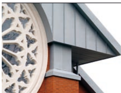
Project: St Georges Church, Catford Architect: Thomas Ford & Partners Installer: Metalex Traditional Metal Roofing Ltd
