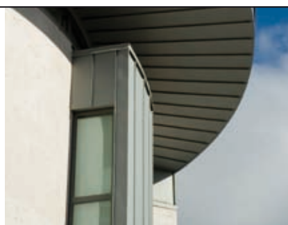
Project: Antrim Civic Centre Architect: W D R & R T Taggart Installer: Longworth Ireland
