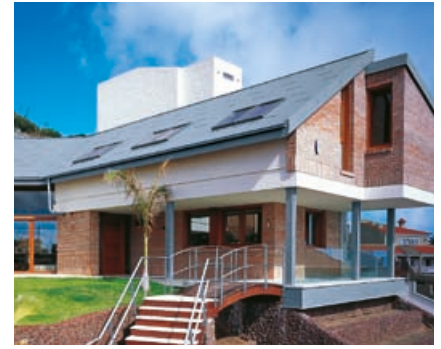
Private Residence Montaña del Socorro, Tafira Baja, Spain
