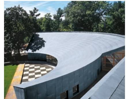
Kaplan Residence, Illinois, USA
