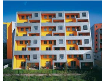
Terrace-shaped building, Oswaldgasse, Vienna, Austria
