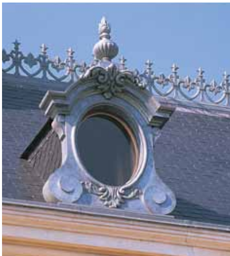
Town Hall, Corbeil-en-Gatinais, France *
