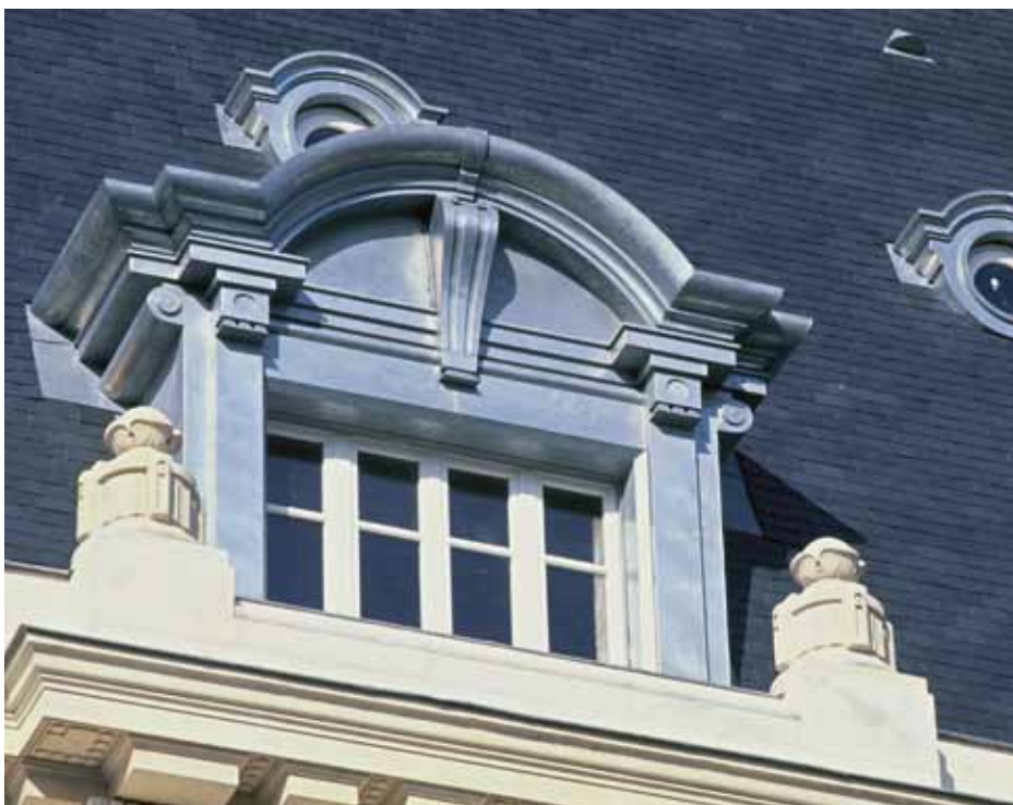
Town Hall, Corbeil Essonnes, France *
