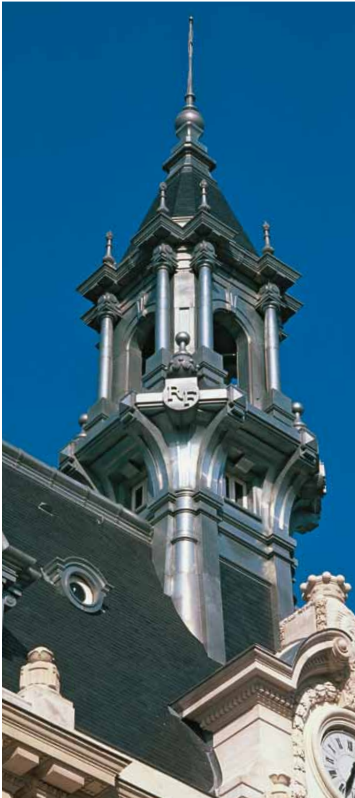
Town Hall, Corbeil-Essonne, France
