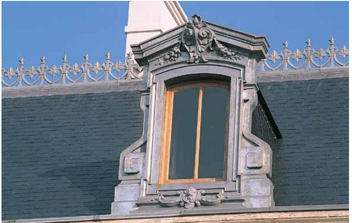
Town Hall, Corbeil-en-Gatinais, France *
