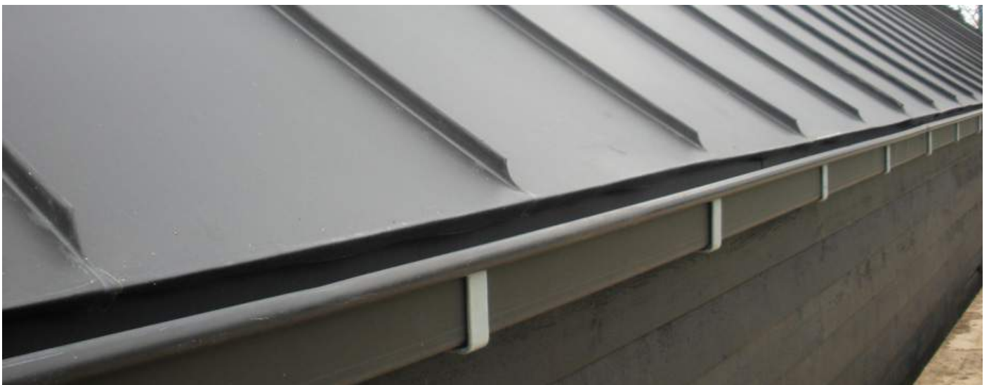
Half Round & Box Gutter Profile
